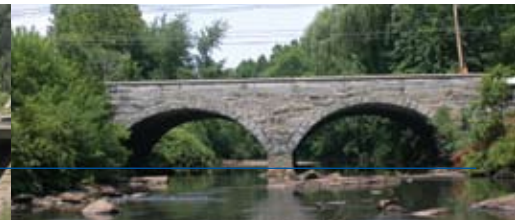
Pont Leominster - Massachusetts
