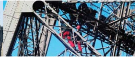
Eiffel Tower - France
