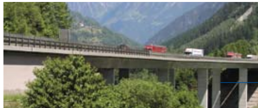
Bridge over the Reuss - Switzerland / Austria
