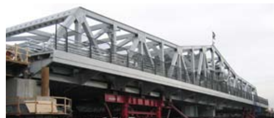
3 rd Avenue Bridge - Manhattan, OSMOS technology during transportation of the bridge
