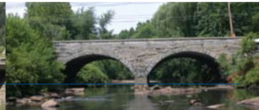
Leominster Bridge - Massachusetts
