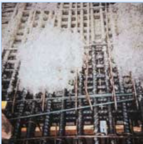
Optical Strand during concrete pouring.
