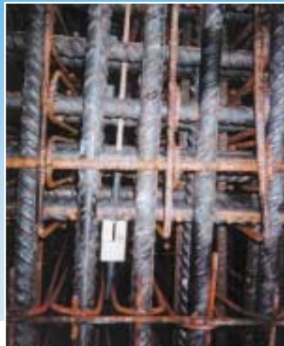
Optical Strand in a reinforcing cage.
